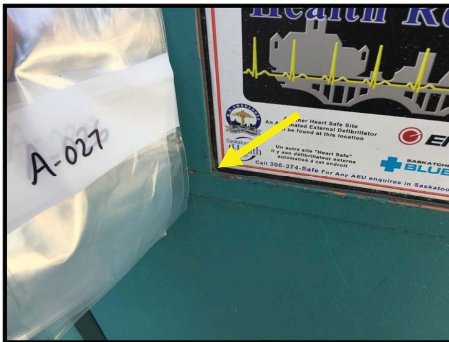
Photograph 1: Asbestos-Containing Black Door Window Caulking.
