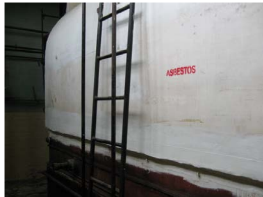
#4) Boiler Insulation
