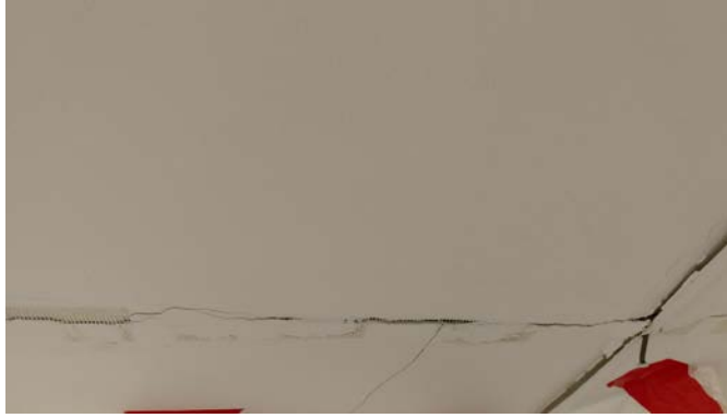
PHOTO 1 – DAY CARE MAIN CORRIDOR – PRIOR TO BULK SAMPLING
