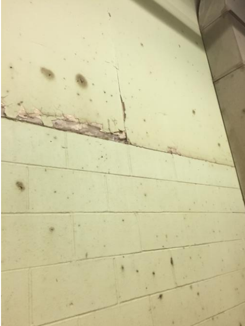
Damaged Drywall
