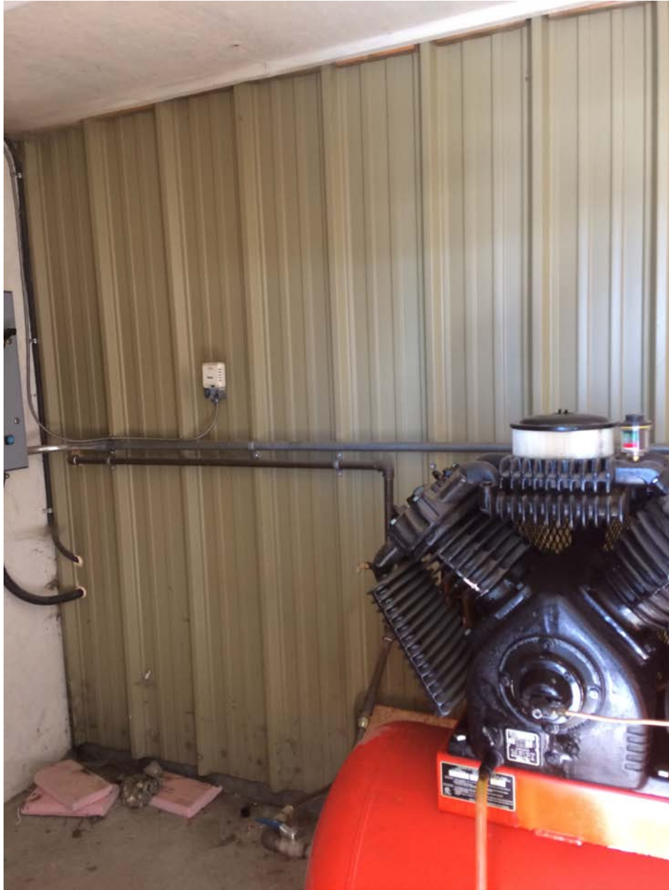
Figure 3- Interior of storage shed.
