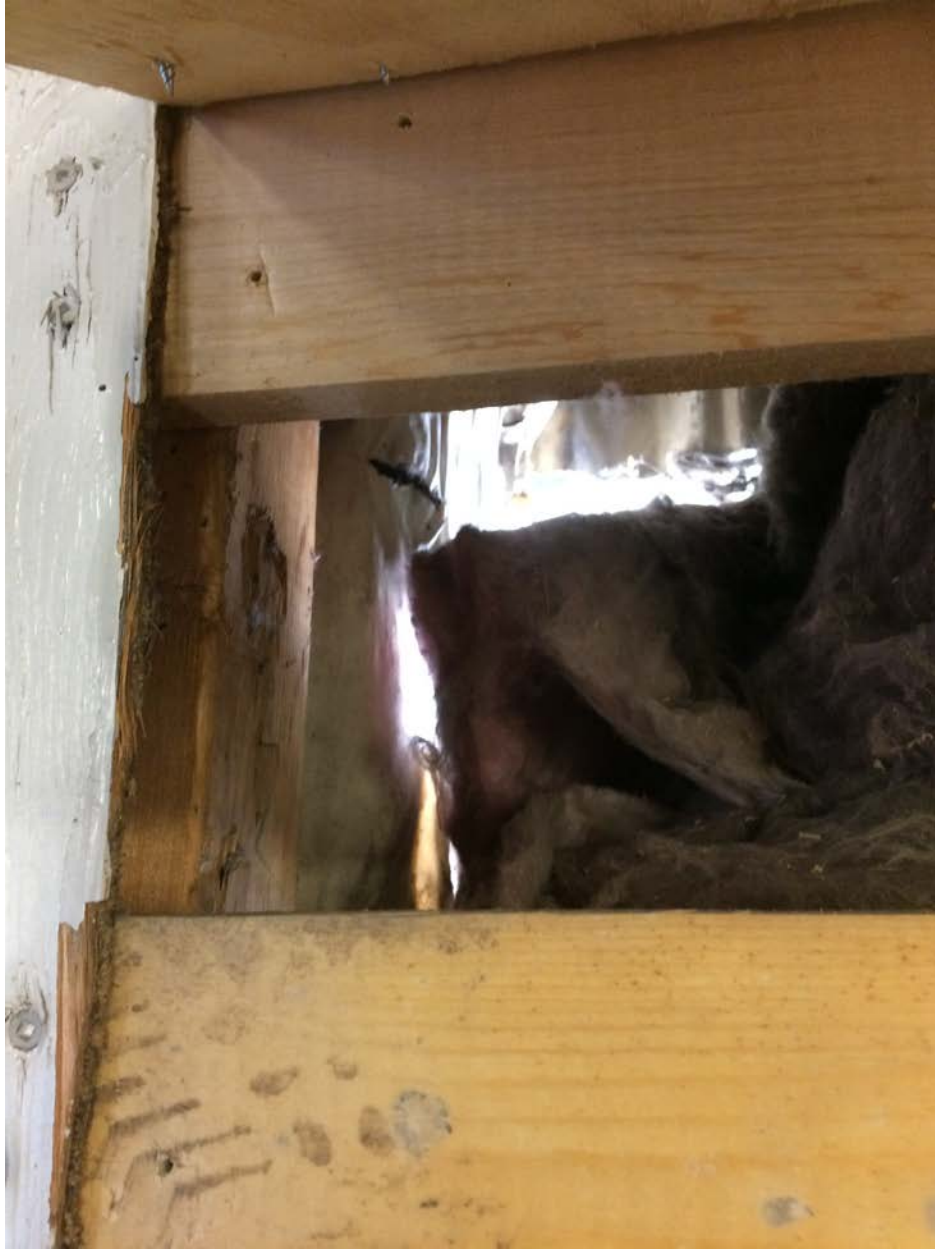
Figure 2- Wall cavity accessed from patch.
