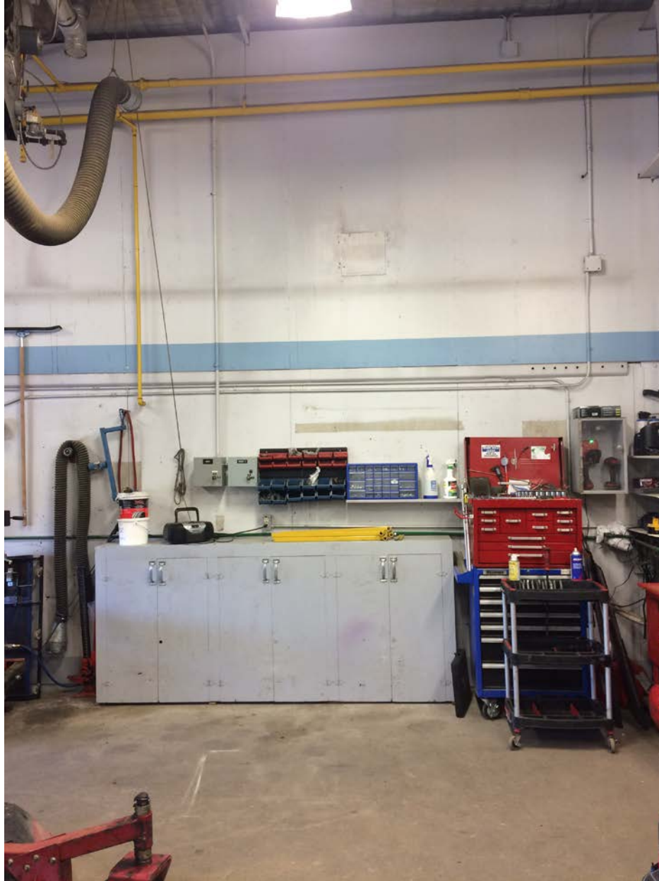
Figure 1- East wall of Maintenance Shop- Lower portion finished with Transite Board.
