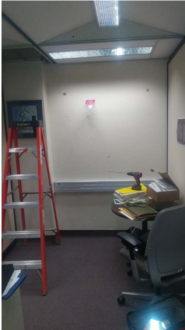
PHOTO 1 – Wall Across from Entrance
