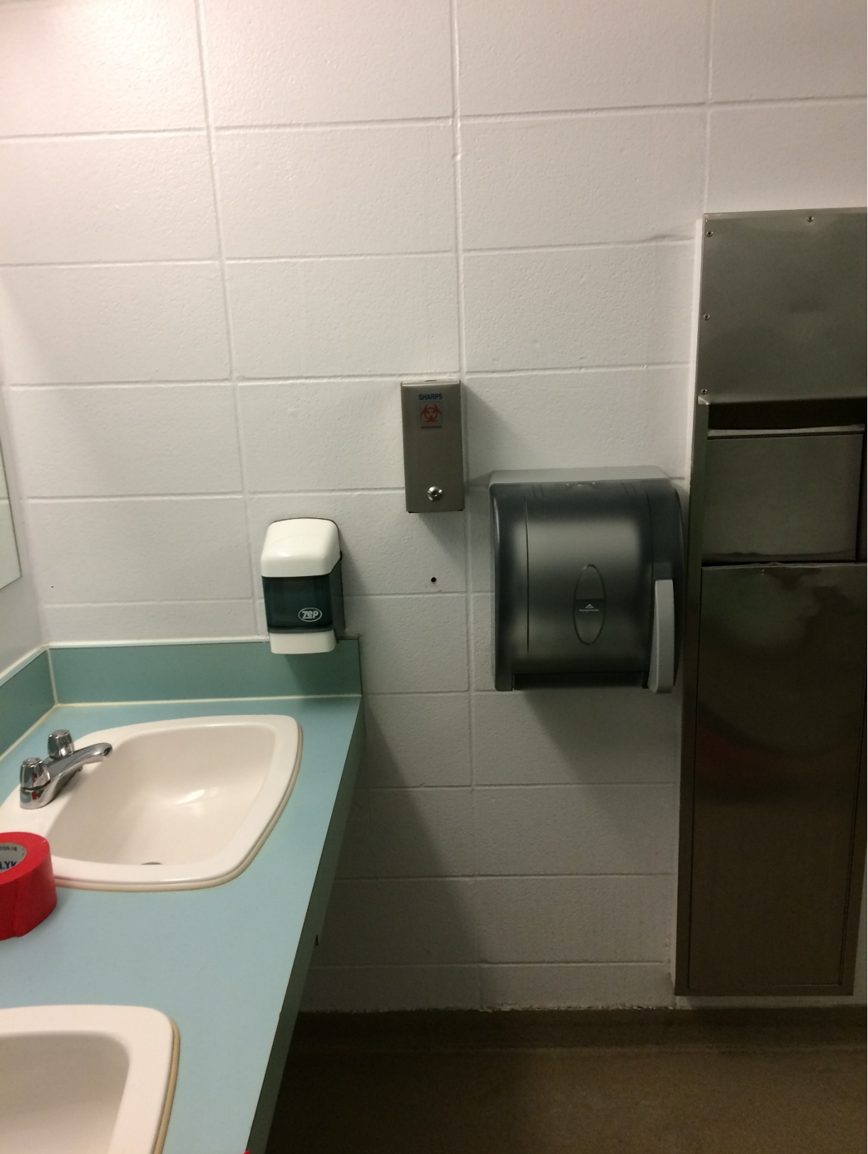
Photo 2- Rm. 146 Men's Washroom
