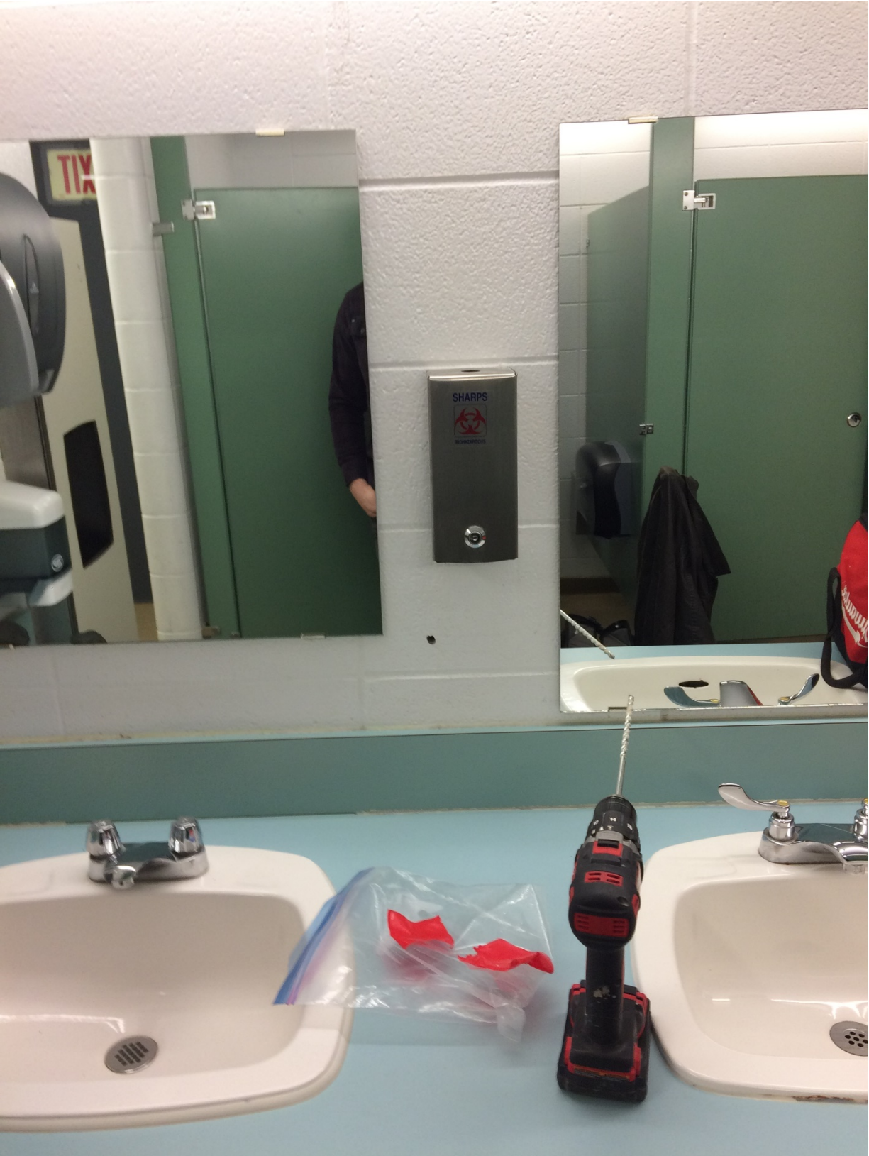
Photo 1- Rm. 152 Men's Changeroom
