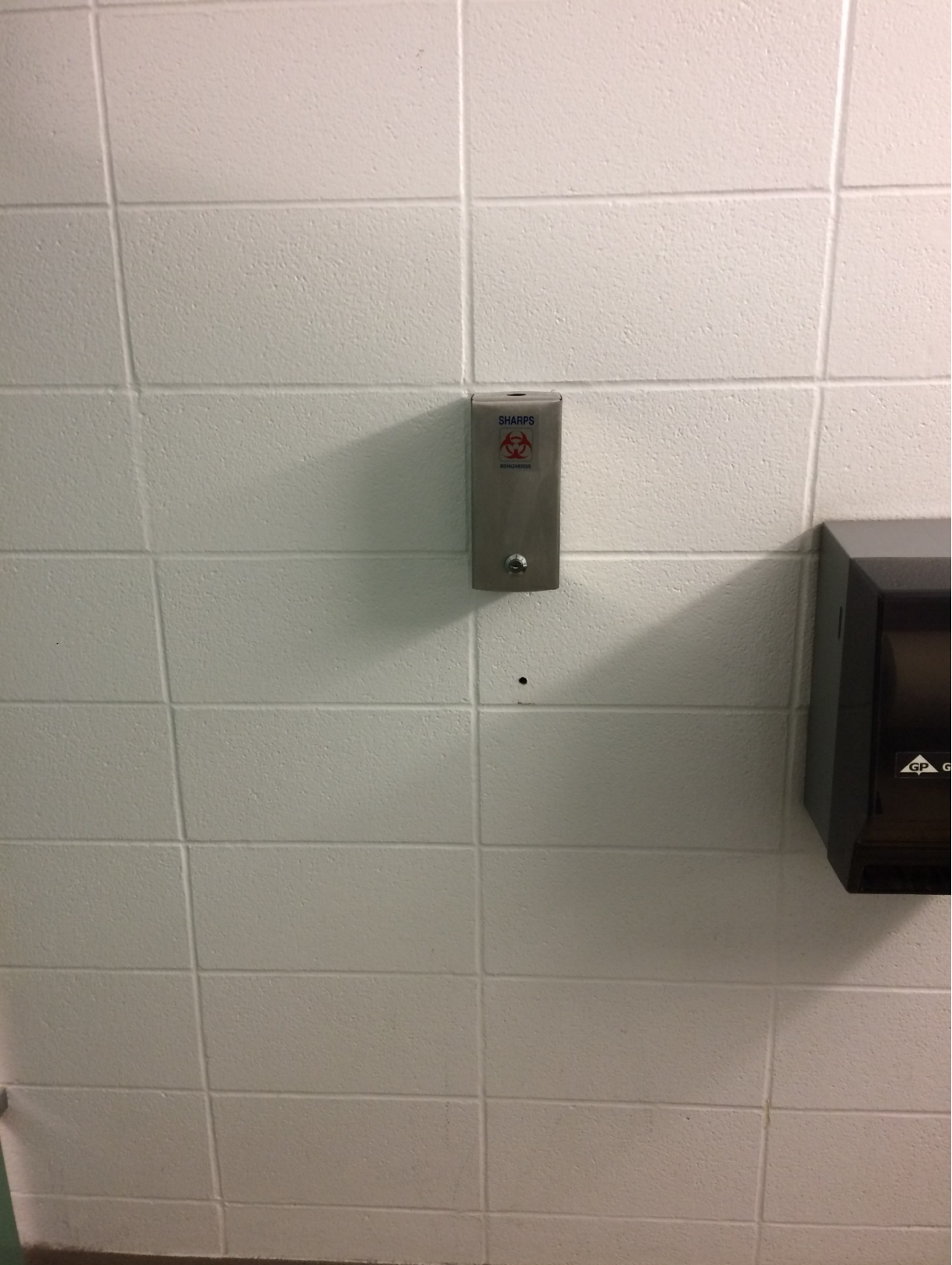
Photo 5- Rm. 217 men's washroom
