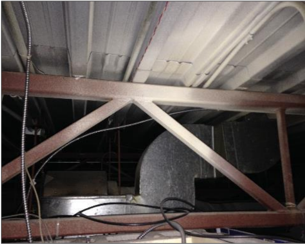
Photo 1: Un-insulated metal duct, structural steel, and metal roof decking above acoustic ceiling tiles in Men's Washroom (Location 105)
