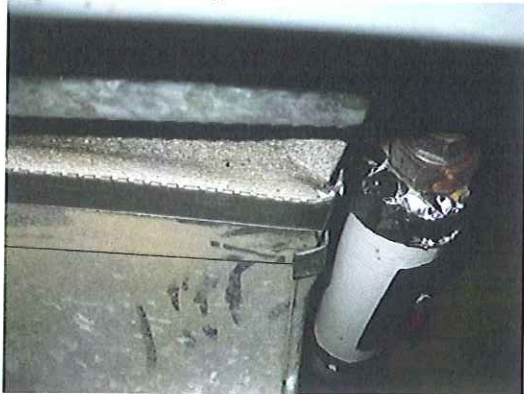
#4) Duct Expansion Gasket
