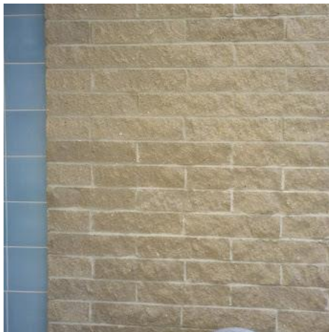
Photo 2: Exterior Brick and Mortar – Adjacent Main Entrance
