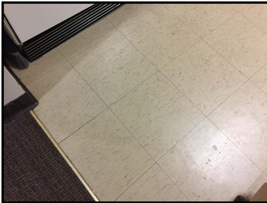
Photograph 1: Asbestos-Containing 12"x12" Beige Floor Tile with Brown Streaks.
