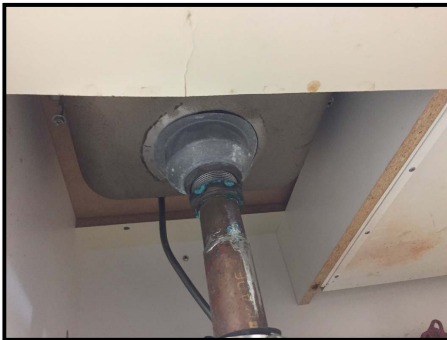
Photograph 2: Asbestos-Containing Gold Sink Undercoat.
