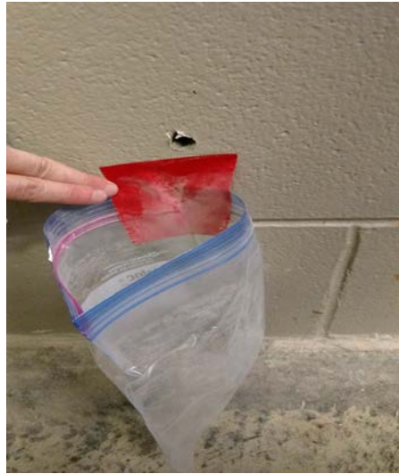
PHOTO 1 – Block Wall Cavity (Empty)
