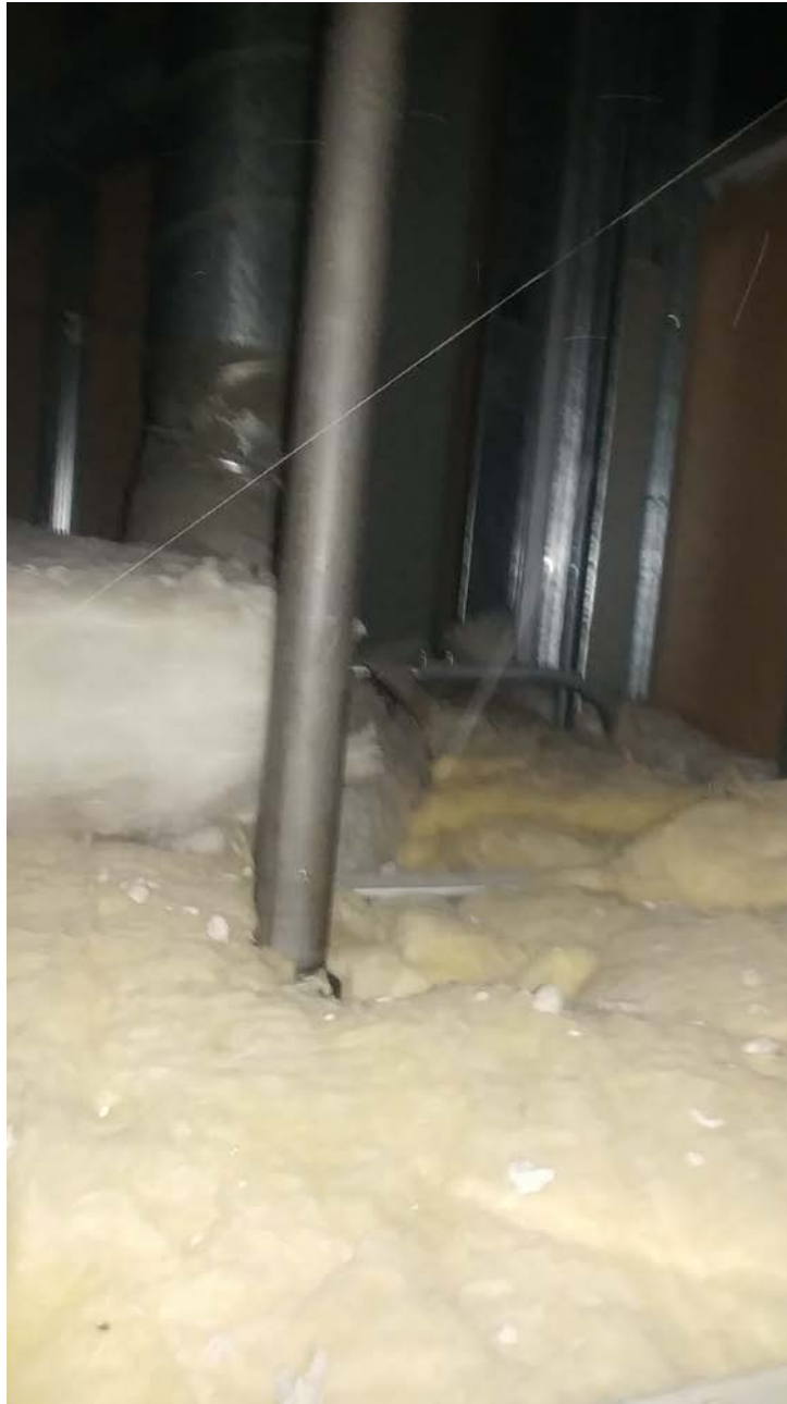
PHOTO 3 – Box Office Washroom Ceiling Space- Fiberglass Insulation
