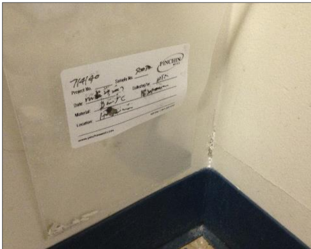
Photo 8 - Drywall Joint Compound on exterior walls (Sample S0003A-C) Hallway Location (117)
