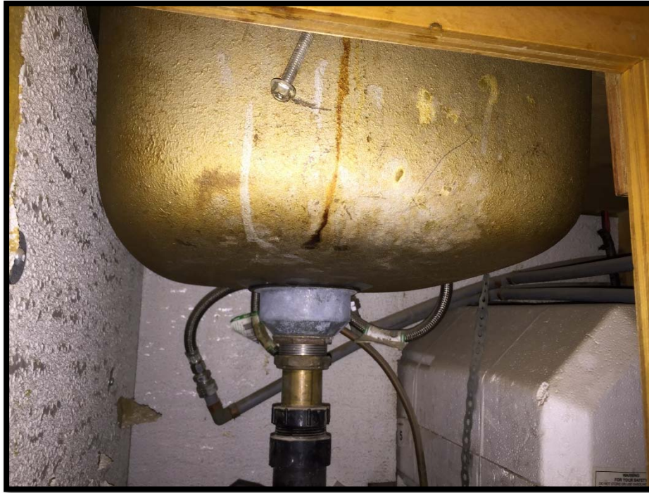
Photograph 1: Asbestos-Containing Gold Sink Undercoat.
