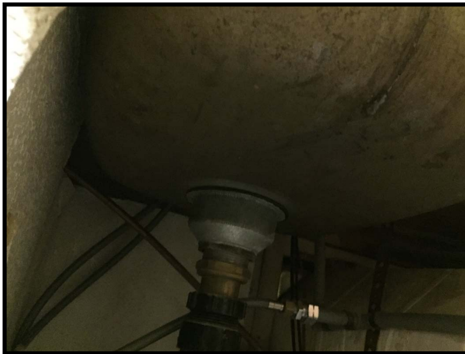
Photograph 1: Asbestos-Containing Silver Sink Undercoat.
