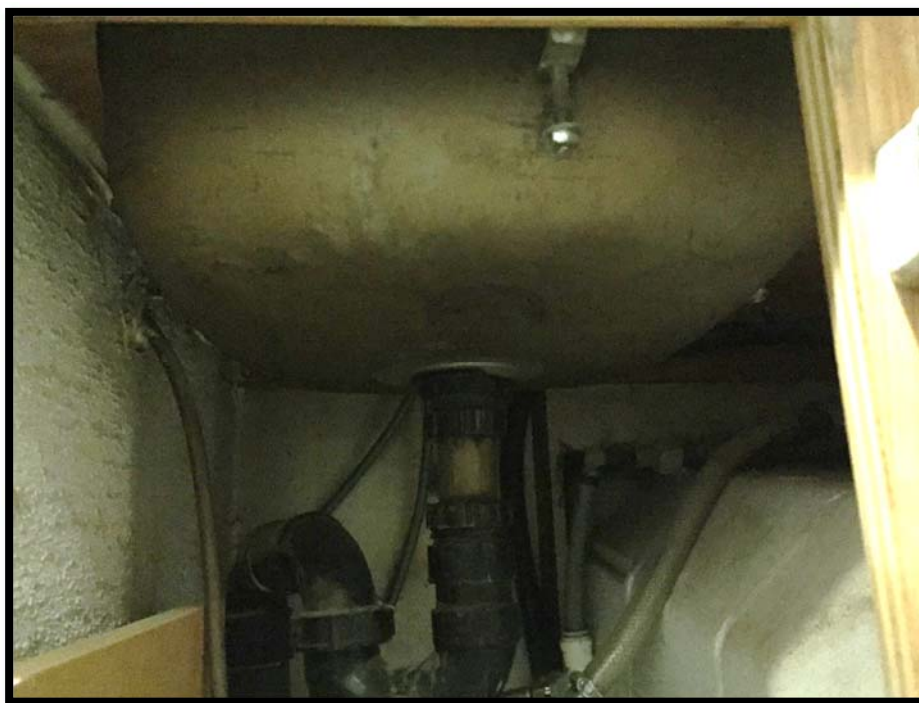
Photograph 1: Asbestos-Containing Gold Sink Undercoat.
