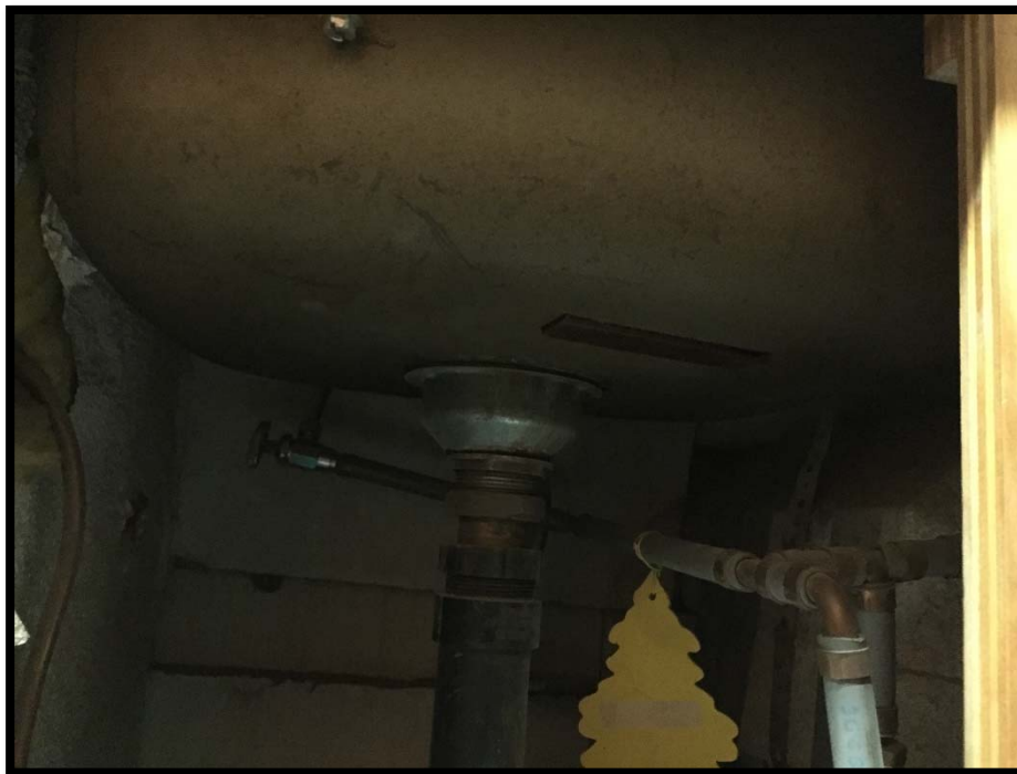
Photograph 1: Asbestos-Containing Gold Sink Undercoat.
