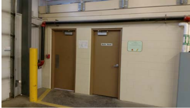
PHOTO 1 – Cindercrete Block Wall
