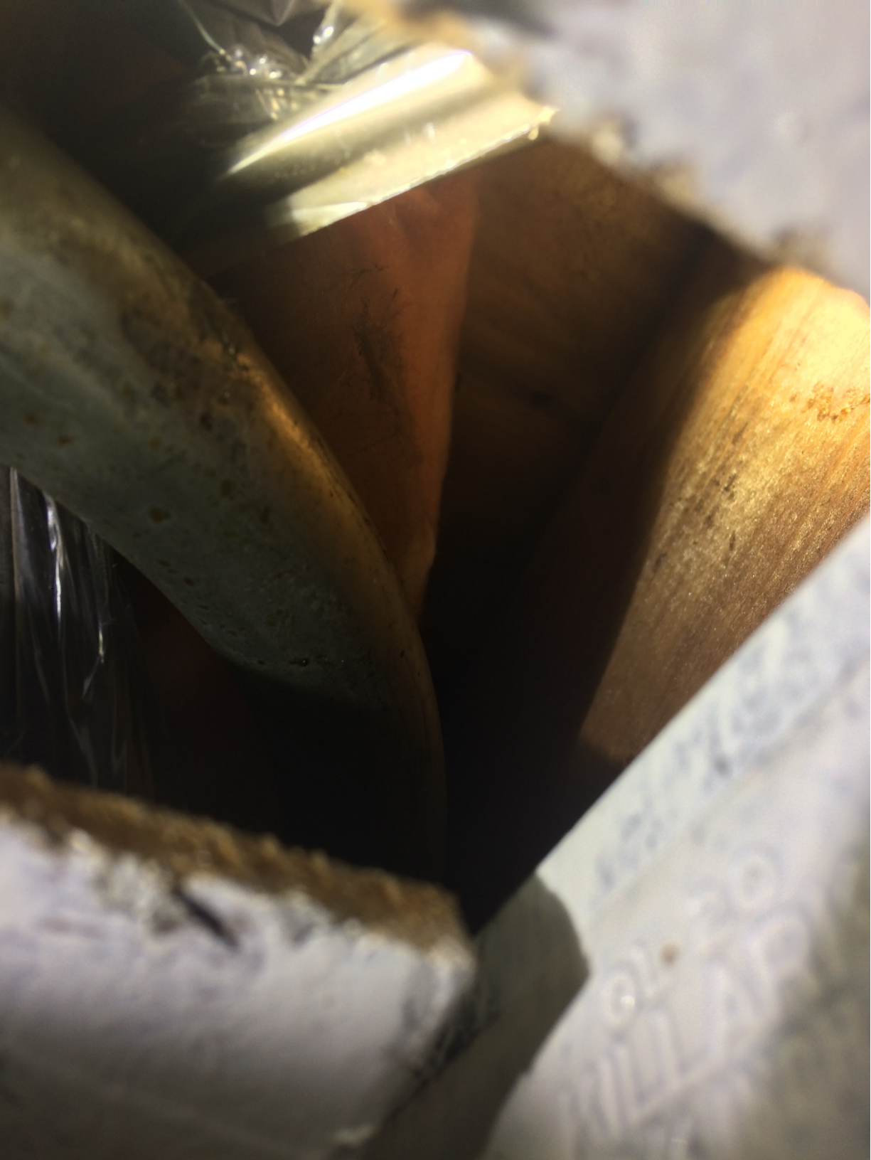
Photo 005- Roof Insulation- Unit 007
