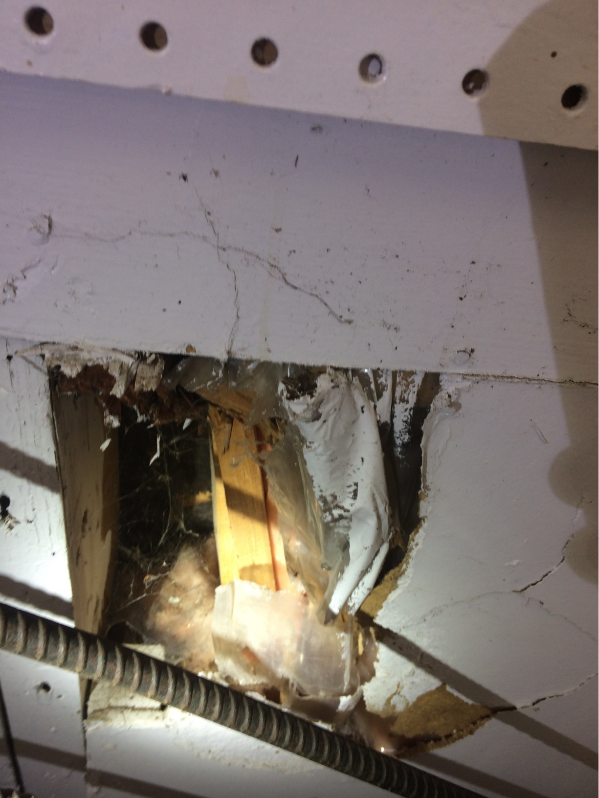
Photo 004- Wall Insulation- Unit 107
