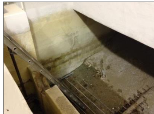
Photo 4– View of white and green lead based paint in a filter tank.
