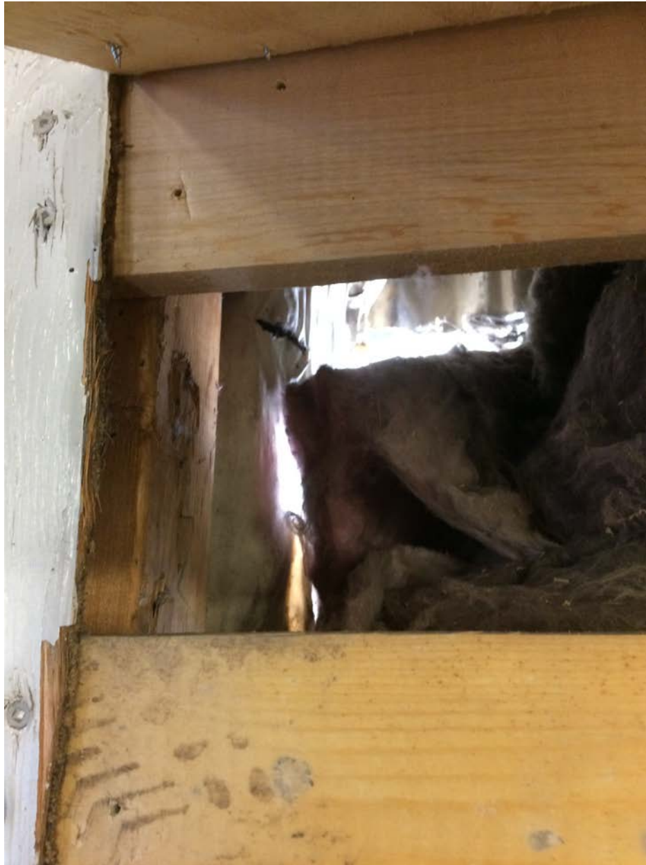
Figure 2- Wall cavity accessed from patch.
