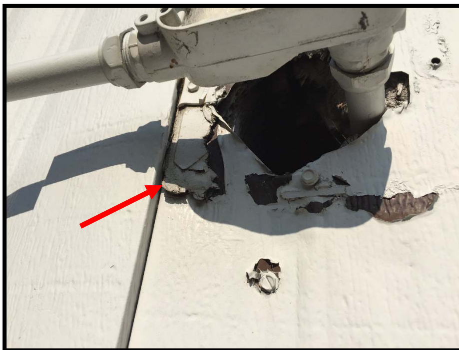
Photograph 1: Asbestos-Containing White Firestop.
