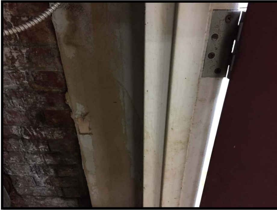
Photograph 7: Asbestos-Containing Drywall Joint Compound.
