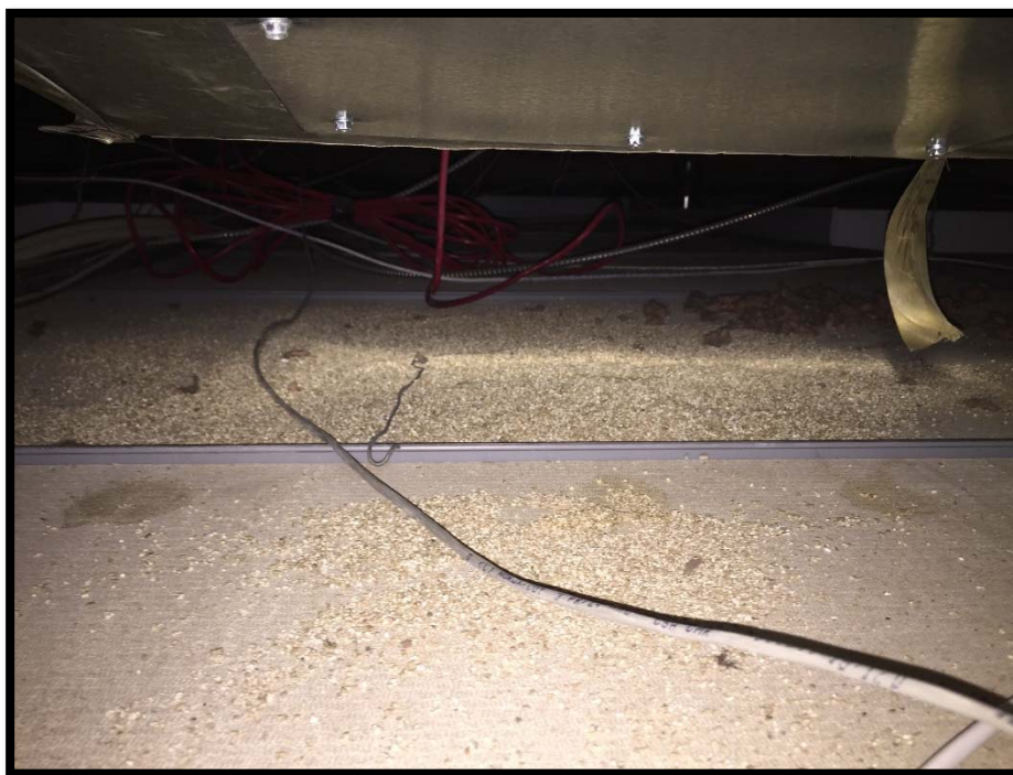
Photograph 10: Suspect Asbestos-Containing Vermiculite Insulation.
