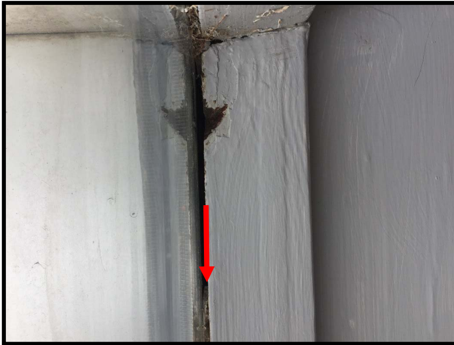
Photograph 6: Asbestos-Containing White Window Caulking.
