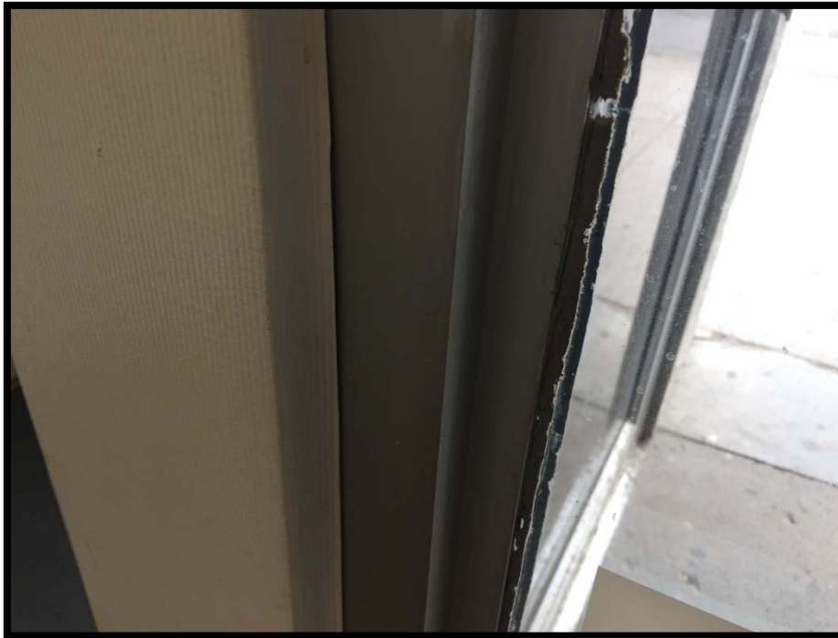
Photograph 8: Asbestos-Containing Grey Window Caulking.
