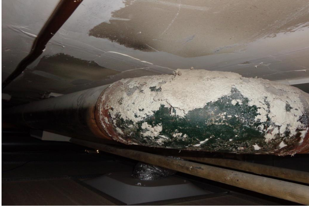
PHOTO 1 – Fire-tape on Drywall Ceiling and Remnants of Asbestos Mud Compound on Pipeline Fitting.
