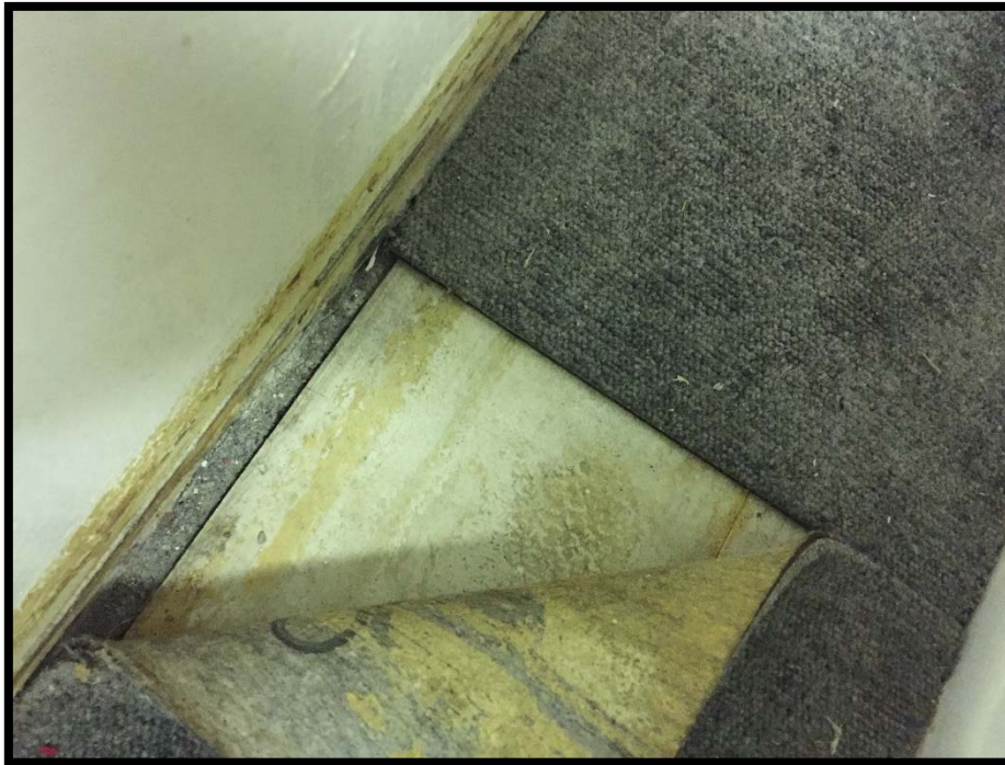
Photograph 2: Asbestos-Containing 12"x12" Floor Tile (Indistinguishable Pattern).
