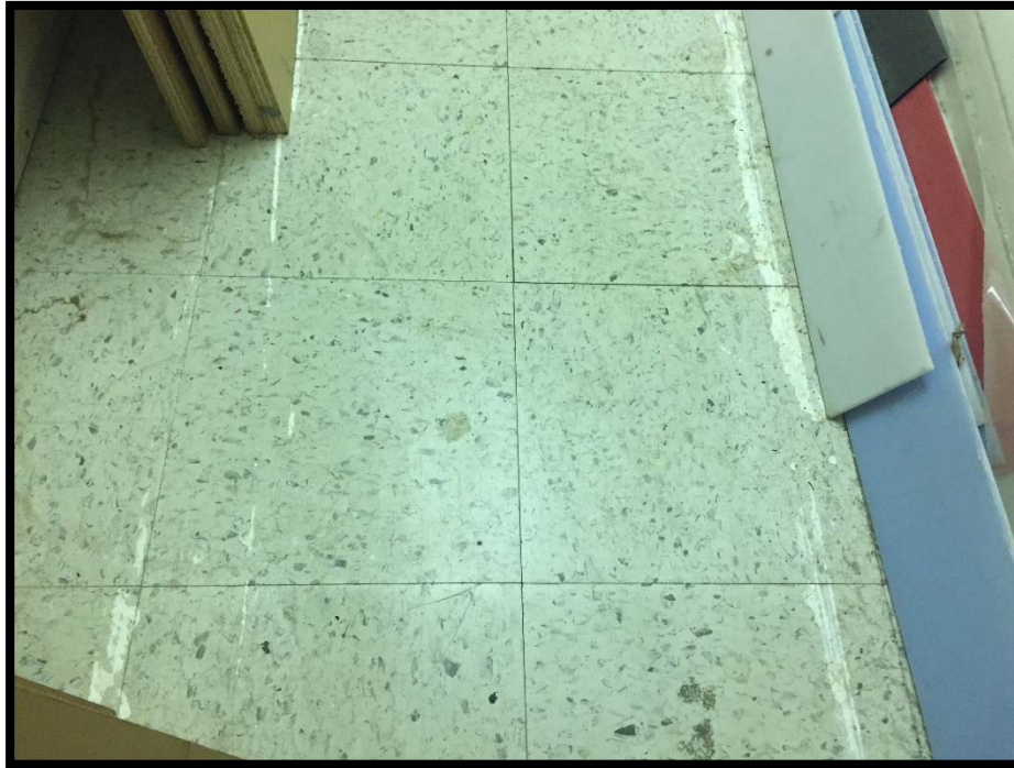
Photograph 1: Asbestos-Containing 12"x12" Off-White Floor Tile with Black Flecks.
