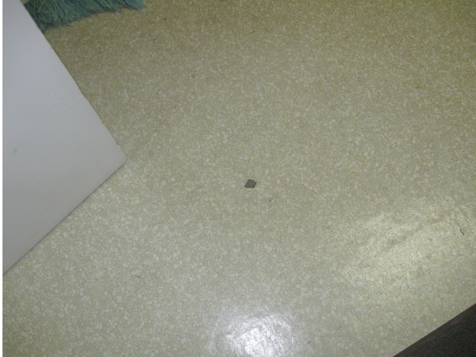
Asbestos Sheet Floor Covering
