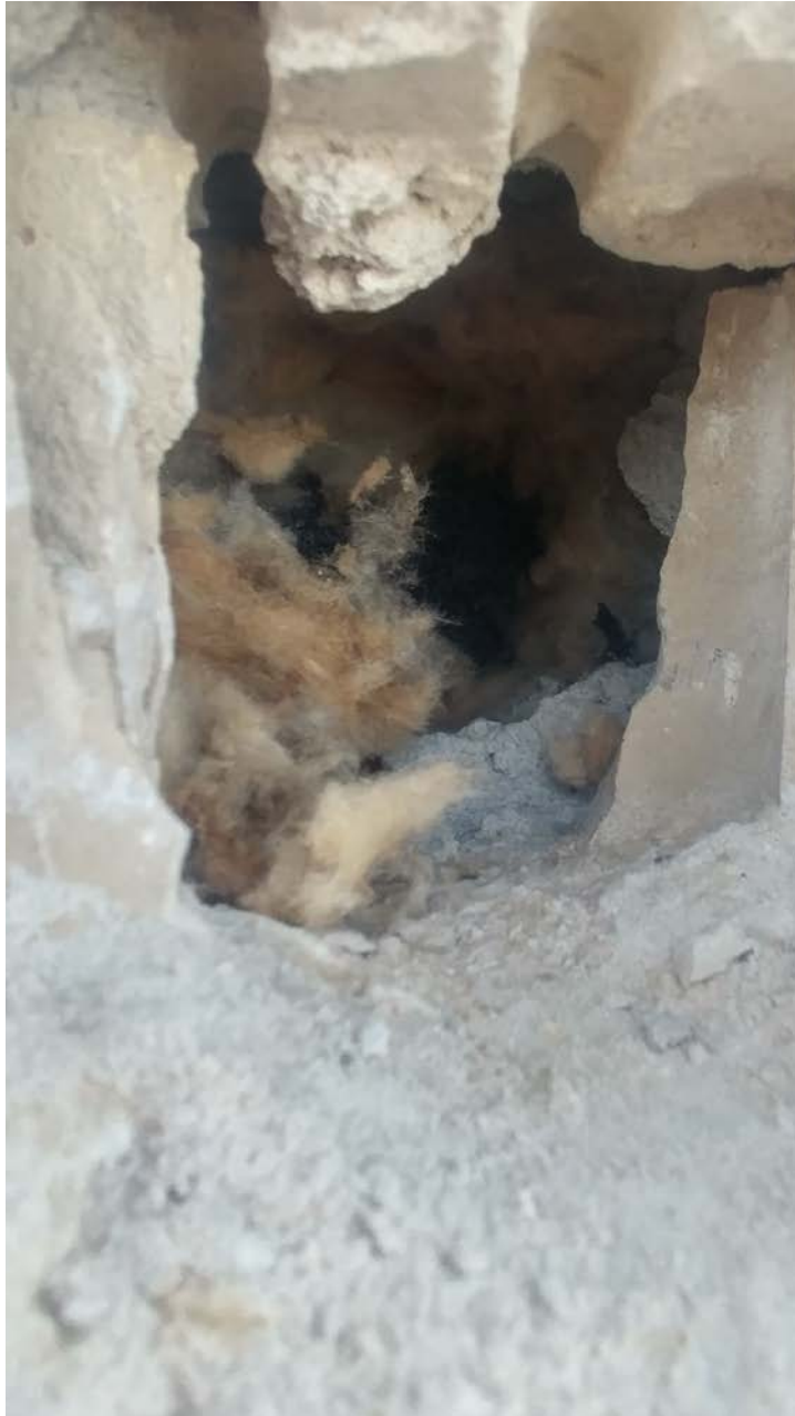
Photo 1- Wall Cavity on Second Floor. (fiberglass insulation)
