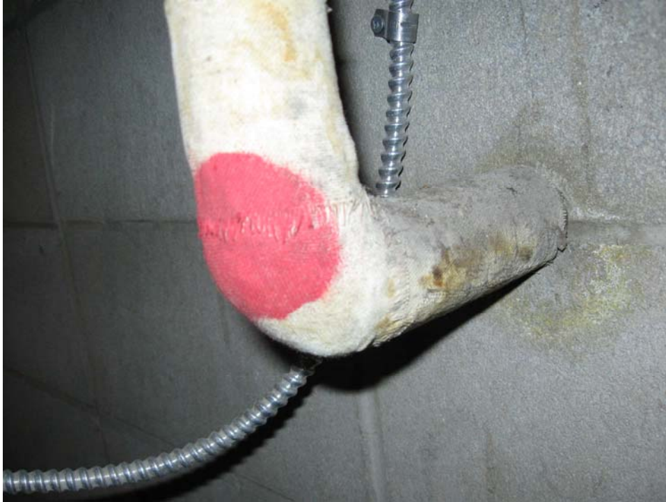
Asbestos Pipeline Fitting (elbow)
