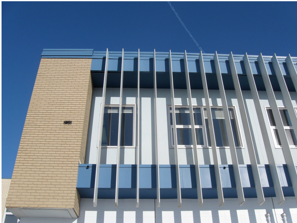
Asbestos Board on wall surface surrounding windows, on the soffit and on the fascia
