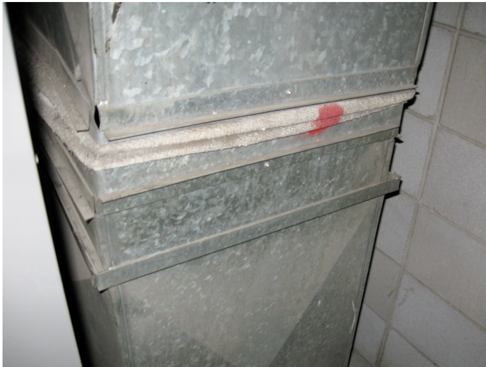
Asbestos Duct Work Woven Expansion Gasket
