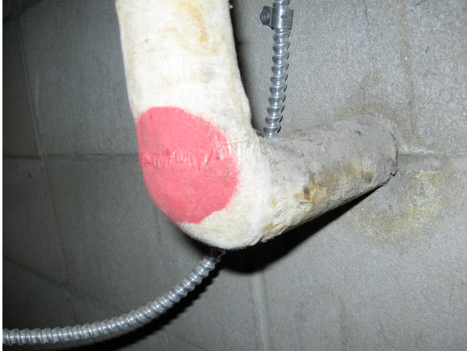
Asbestos Pipeline Fitting (elbow)
