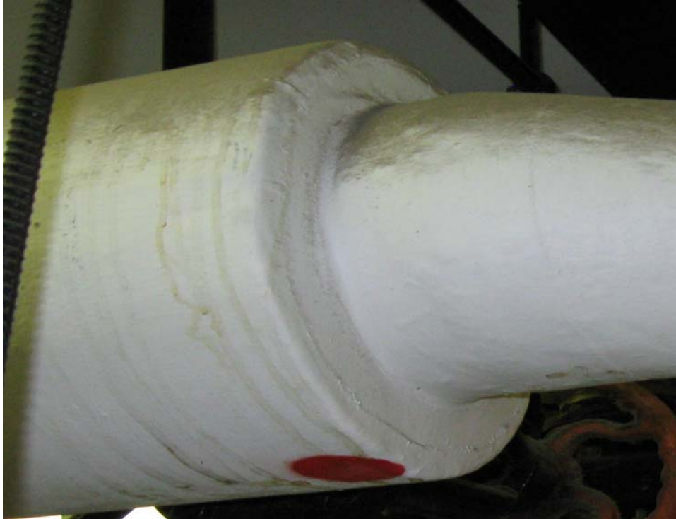
Asbestos Mud Compound on mechanical pipeline end cap
