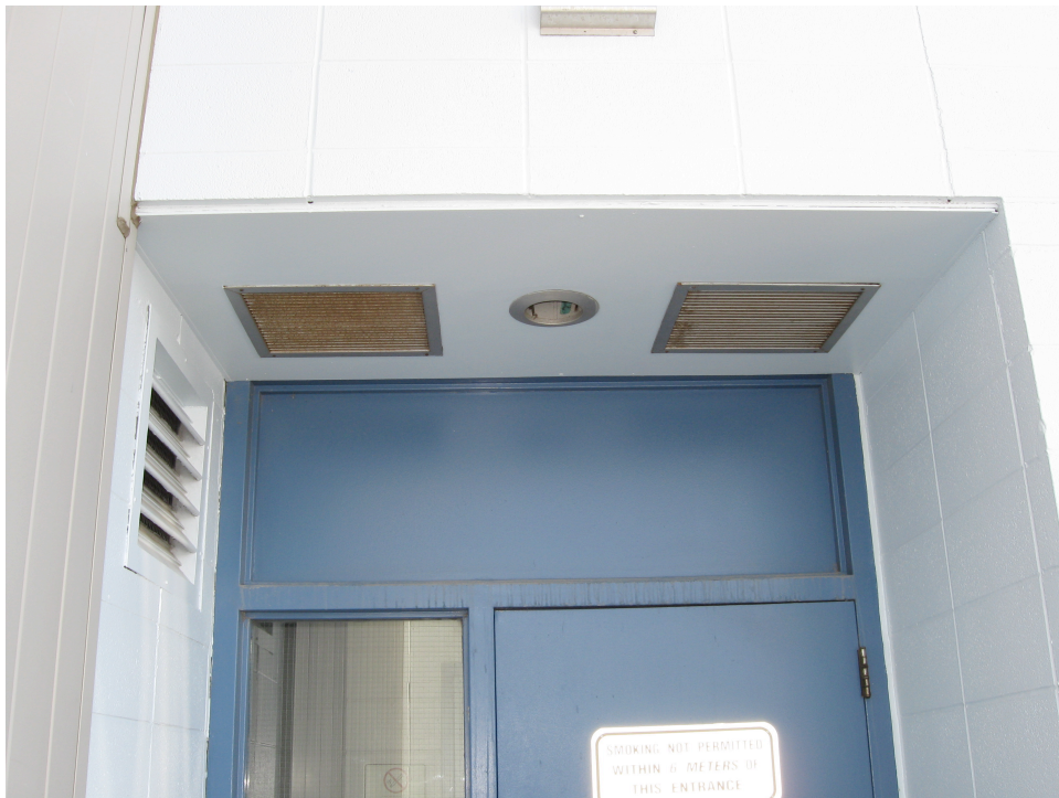
Asbestos Board above doorways
