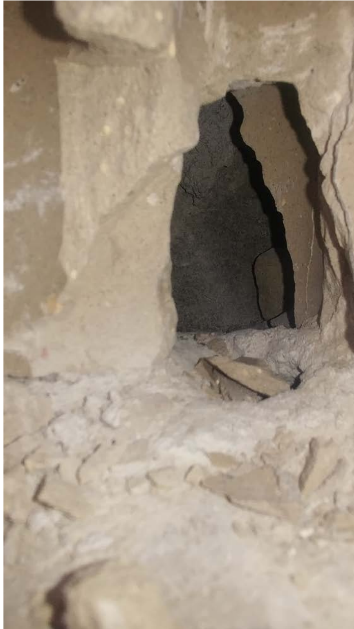
Photo 2- Wall Cavity in Lower Section
