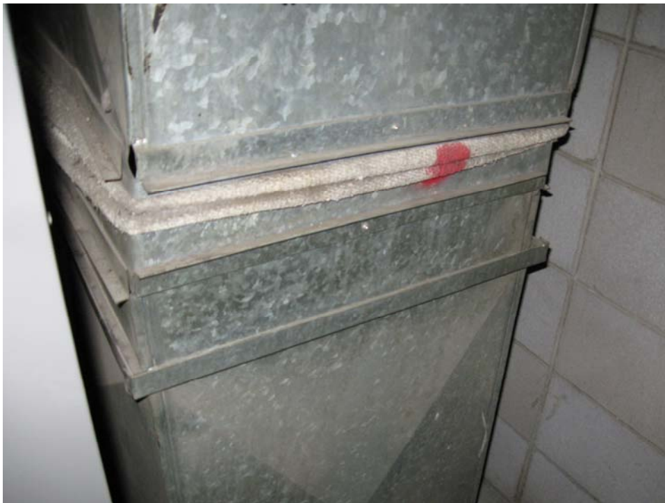
Asbestos Duct Work Woven Expansion Gasket
