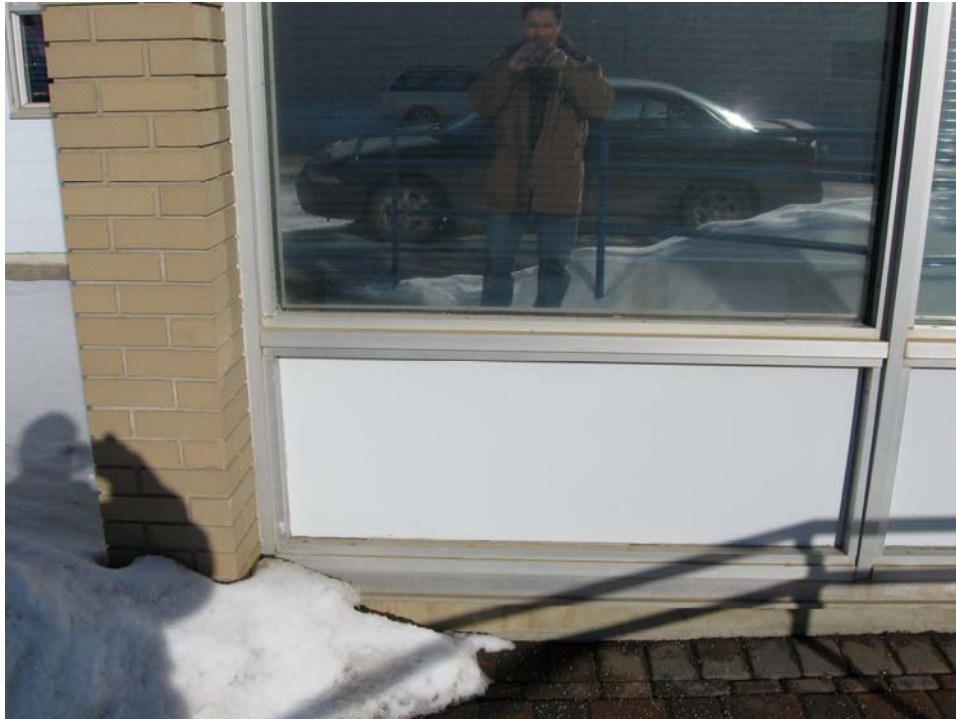
Asbestos Board below main entry windows
