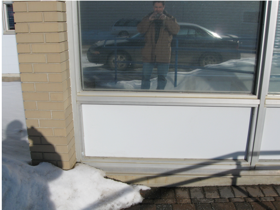
Asbestos Board below main entry windows
