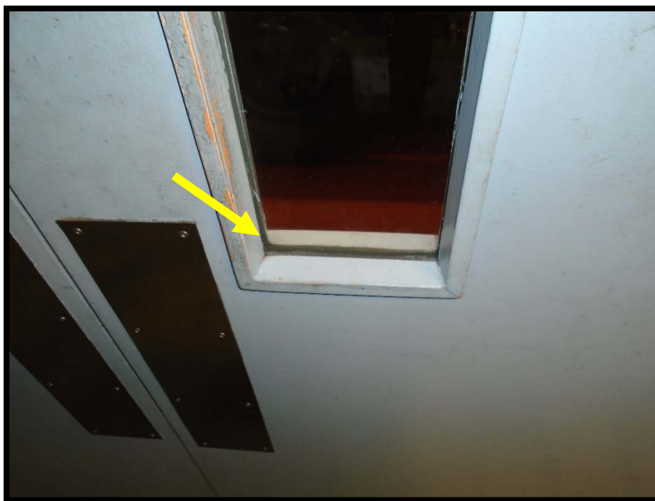
Photograph 1: Asbestos-Containing Grey Window Caulking.
