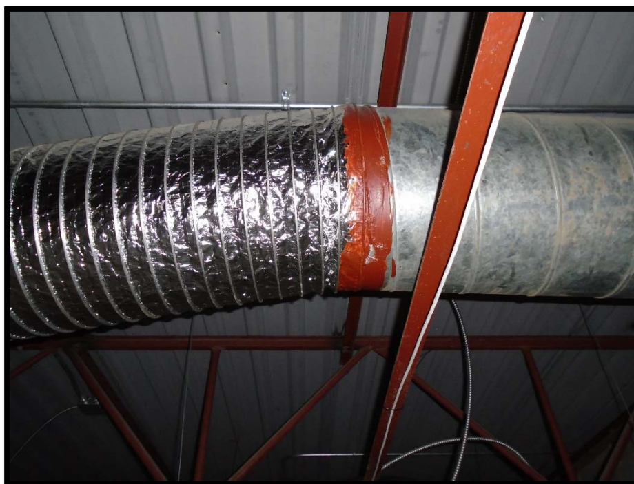
Photograph 2: Asbestos-Containing Red/Brown Duct Mastic.
