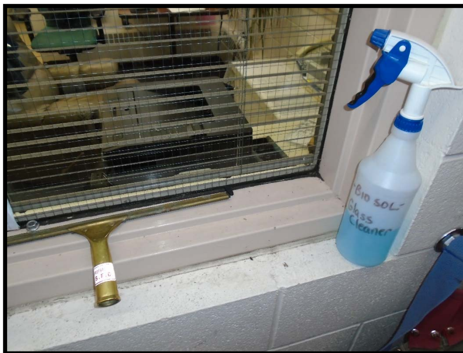
Photograph 1: Asbestos-Containing Black Window Caulking.
