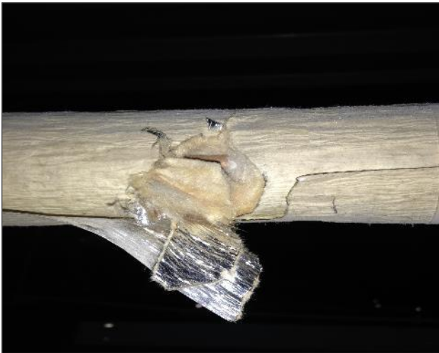
Photo 1 - Non-Asbestos containing fiberglass piping insulation on piping above acoustic ceiling tiles in boardroom
