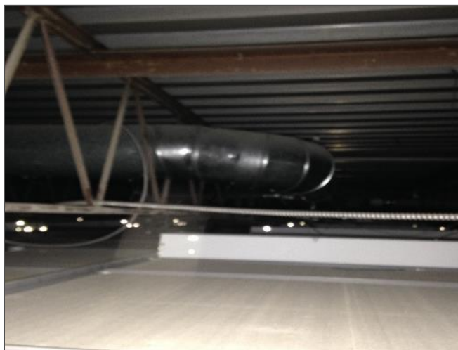
Photo 3: Un-insulated metal duct, structural steel roof truss, and metal roof decking above acoustic ceiling tiles in training room.
