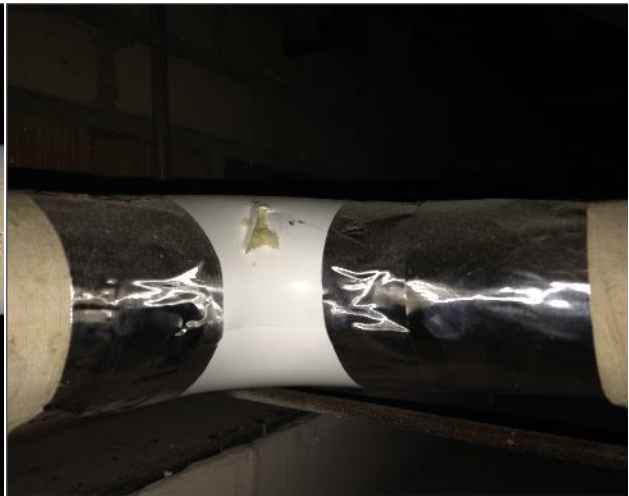
Photo 2 - Non-Asbestos containing fiberglass piping insulation on pipe elbows above acoustic ceiling tiles in boardroom.
