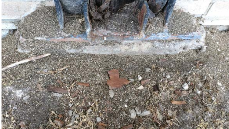
PHOTO 1 – Exterior Brick Wall
