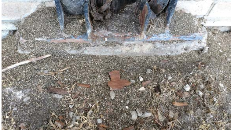
PHOTO 1 – Exterior Brick Wall
