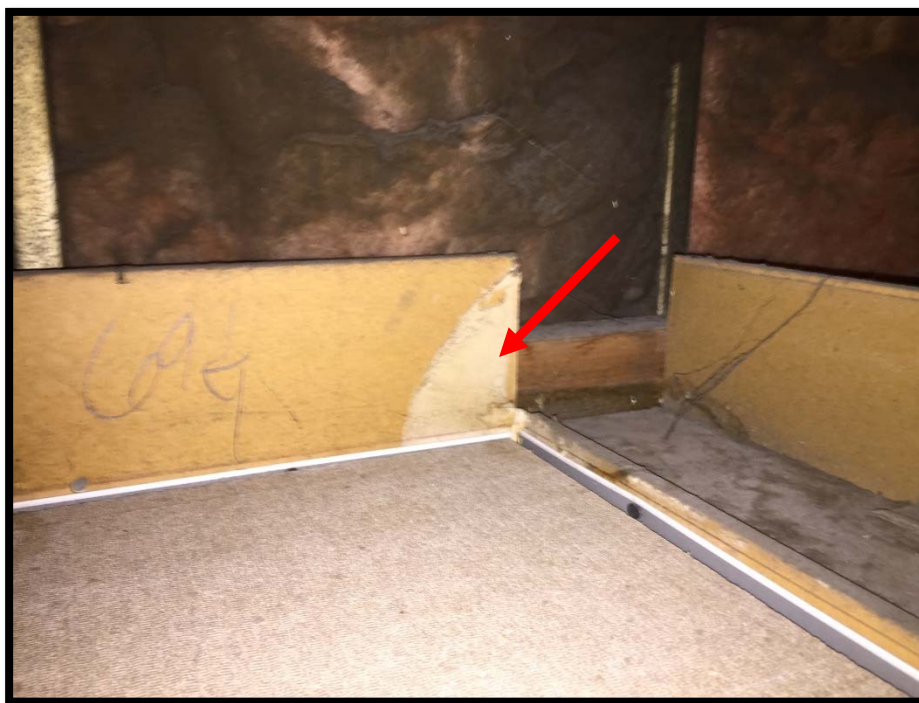
Photograph 3: Asbestos-Containing Drywall Joint Compound.
