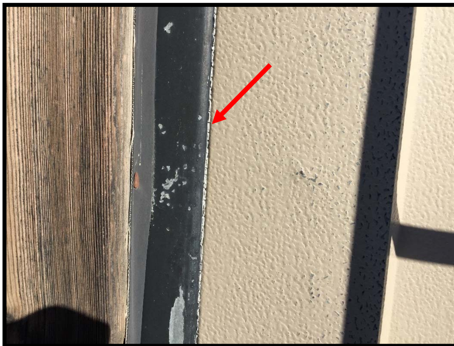
Photograph 2: Asbestos-Containing White Overhead Door Caulking.
