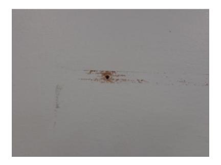
**AREA 6:** First Level – Room 118, No Asbestos Detected on North Wall Surface Where the Conduit is Mounted to. The Surface Consists of Painted 3/8" Plywood.
