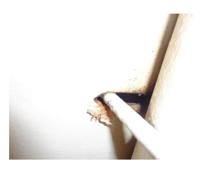
**AREA 5:** First Level – Room 112, No Asbestos Detected on West Wall Surface Where the Projector Screen is Mounted to. The Surface Consists of Painted 3/8" Plywood.
