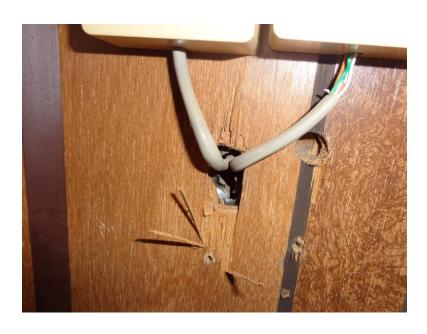
**AREA 13:** Second Level – Room 35B West Upper Wall. The Surface Consists of Painted 3/8" Plywood, an Empty Wall Cavity and 3/8" Plywood on the Opposite Side of the Wall (236A Corridor).
