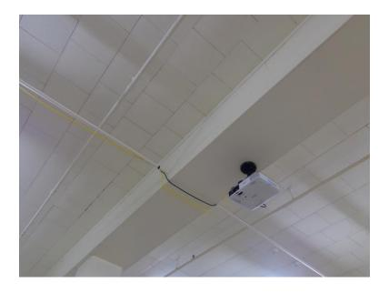
**AREA 4:** First Level – Room 112, No Asbestos Detected in Bulk Head Surface. This Photo is at the Pipe Hanger to the South of the Projector. The Surface Consists of Painted 3/8" Plywood.
