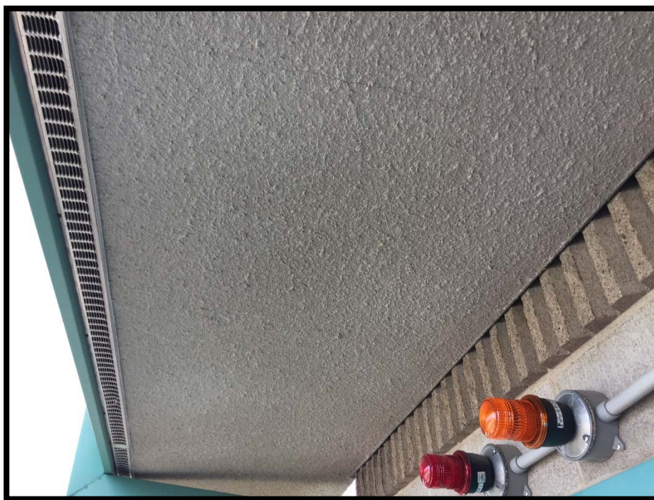
Photograph 1: Asbestos-Containing Concrete Texture Coat.
