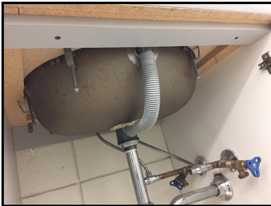
Photograph 2: Asbestos-Containing Gold Sink Undercoat.
