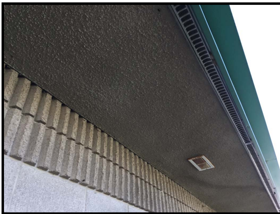
Photograph 1: Asbestos-Containing Concrete Texture Coat.
