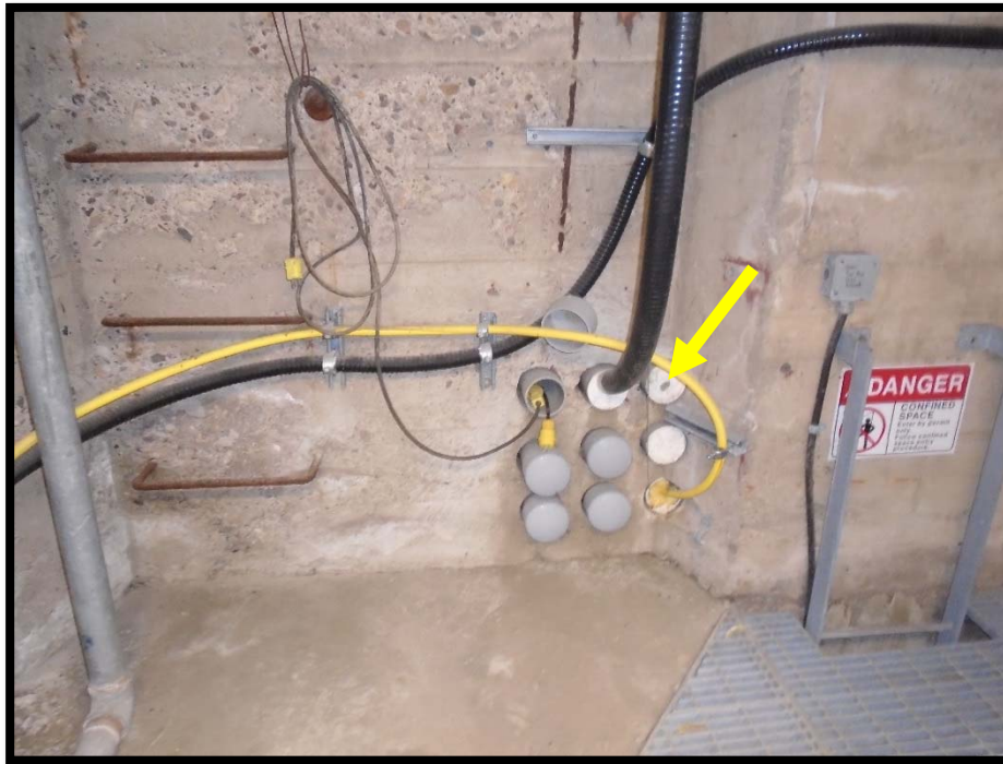
Photograph 3: Asbestos-Containing Yellow Insulation Inside Cable Conduit, Behind White Firestop
