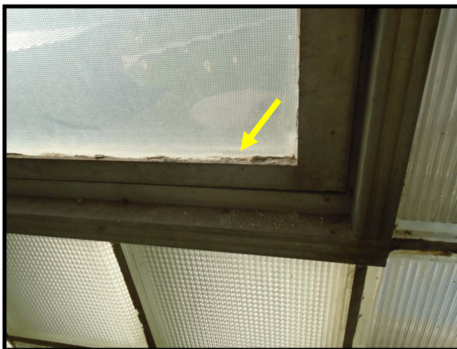
Photograph 2: Asbestos-Containing Grey Window Glazing Below White Caulking.
