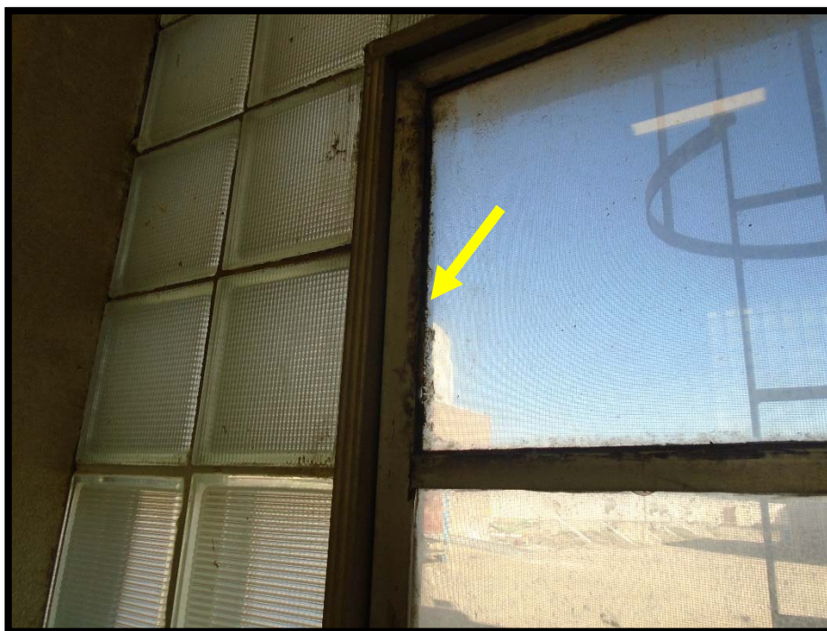
Photograph 1: Asbestos-Containing Black Window Glazing.
