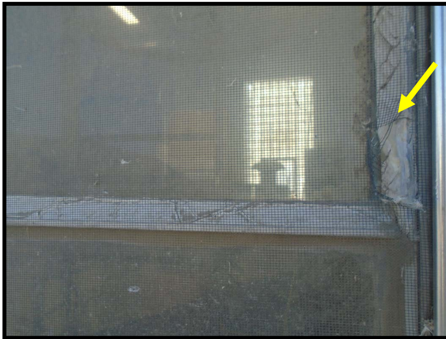
Photograph 4: Asbestos-Containing Exterior White Caulking on Window Pane
