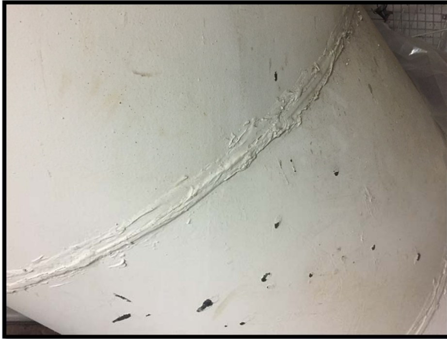
Photograph 1: Asbestos-Containing Tan Duct Mastic (Painted White).
