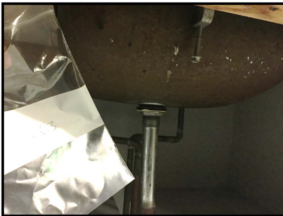
Photograph 3: Asbestos-Containing Gold Sink Undercoat.
