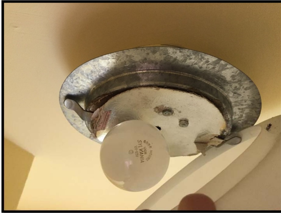
Photograph 3: Asbestos-Containing Incandescent Light Fixture Paper.
