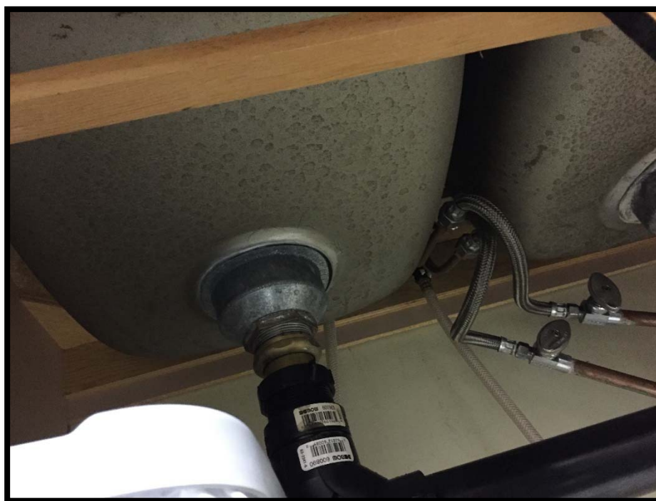
Photograph 2: Asbestos-Containing Silver Sink Undercoat.
