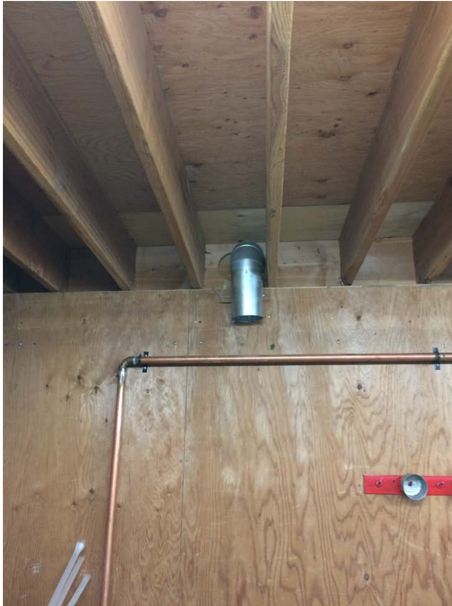
Figure 2- Exterior wall of storage room showing existing vent to be used.
