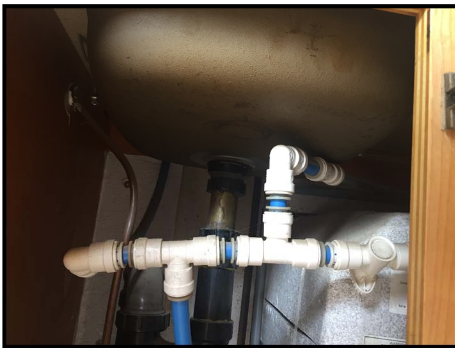
Photograph 1: Asbestos-Containing Gold Sink Undercoat.
