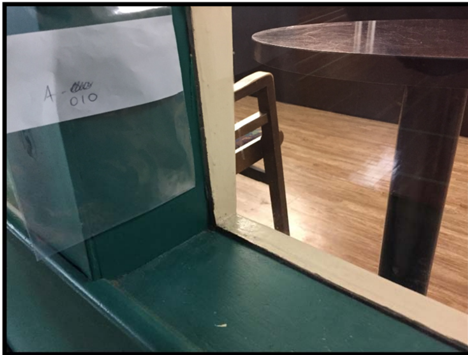
Photograph 2: Asbestos-Containing Black Window Caulking.
