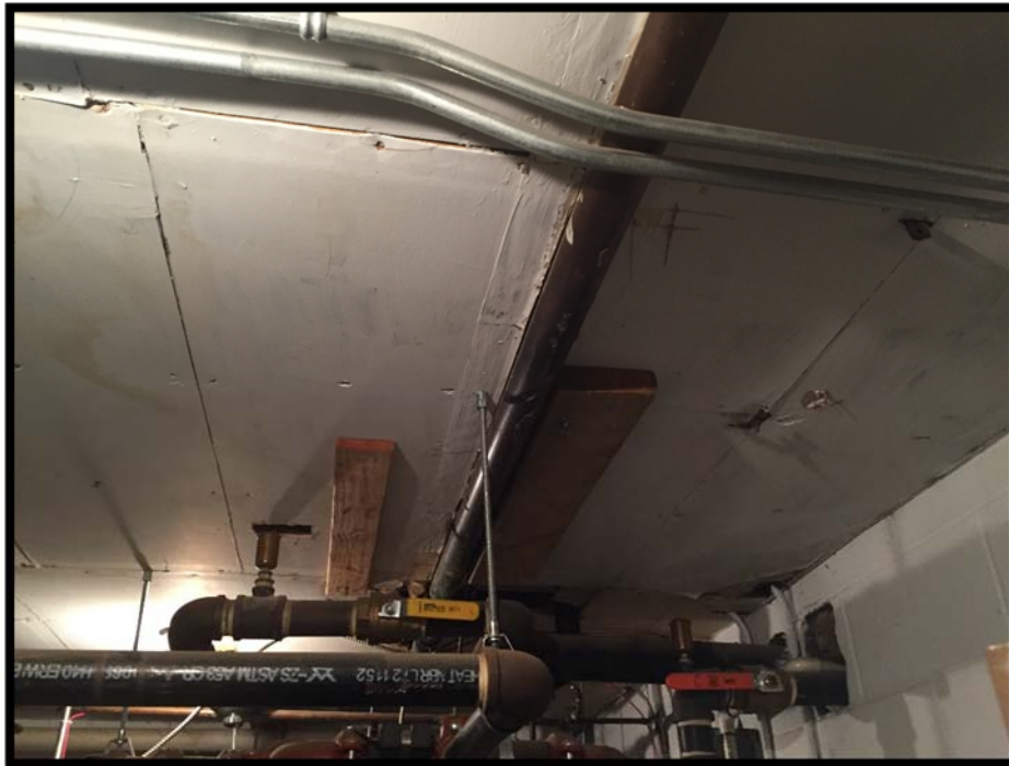
Photograph 1: Asbestos-Containing Drywall Joint Compound.
