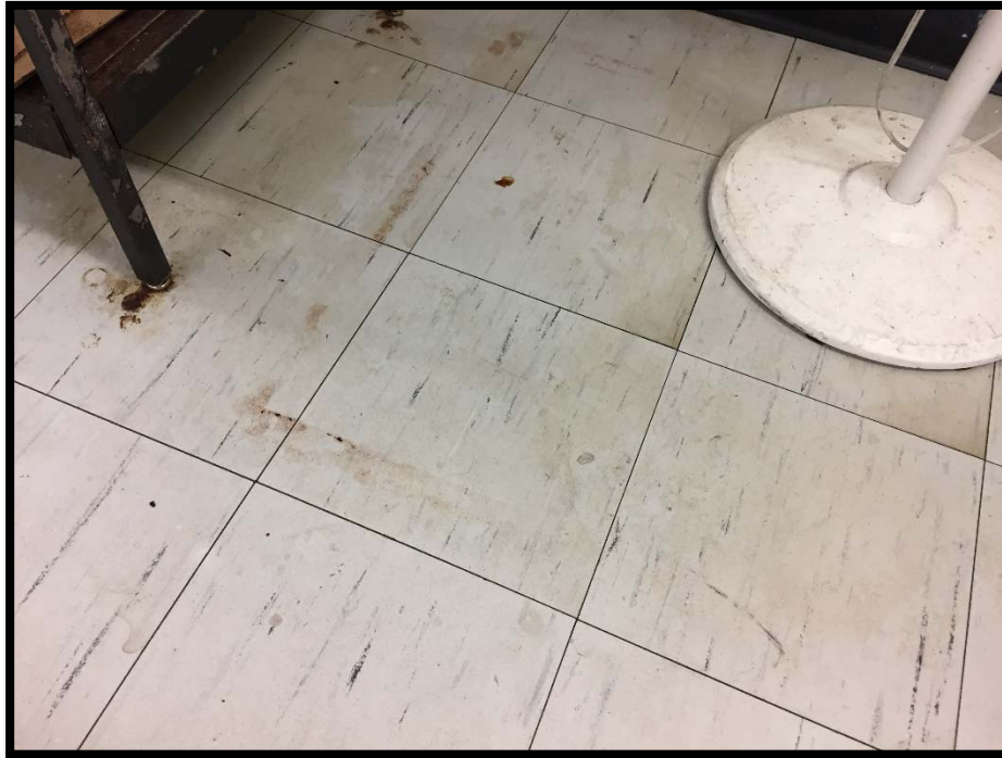
Photograph 1: Asbestos-Containing 12"x12" Off-White Floor Tile with Black Streaks.
