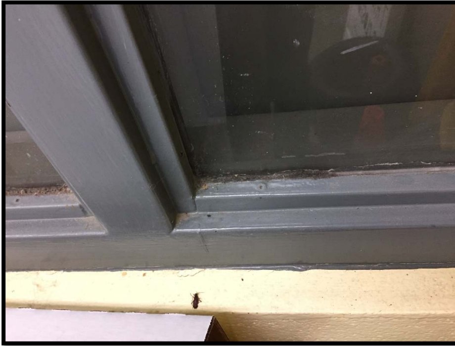
Photograph 3: Asbestos-Containing Grey Window Caulking.
