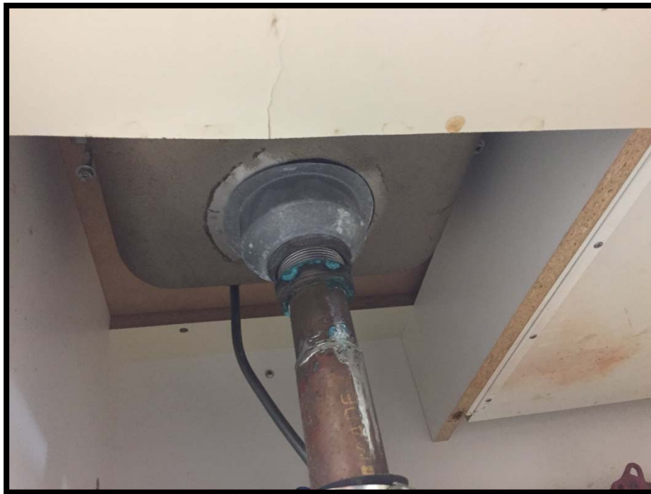
Photograph 2: Asbestos-Containing Gold Sink Undercoat.
