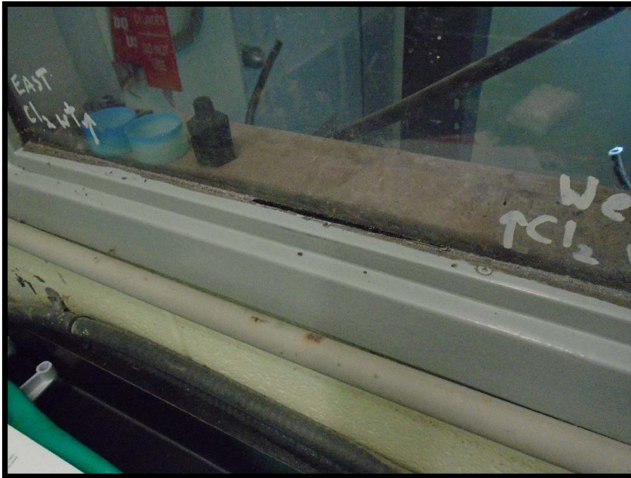
Photograph 4: Asbestos-Containing Black Window Putty.
