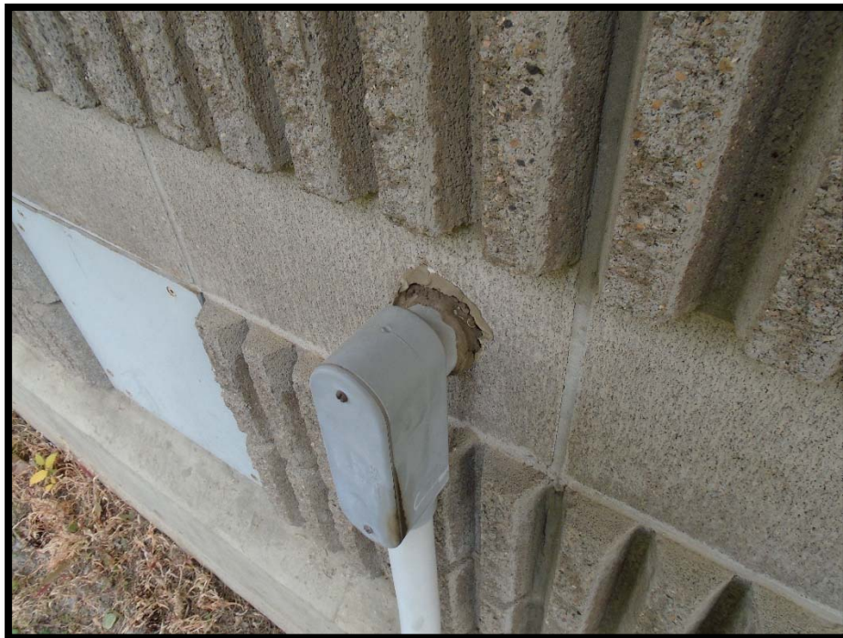
Photograph 6: Asbestos-Containing Light Grey Building Caulking.
