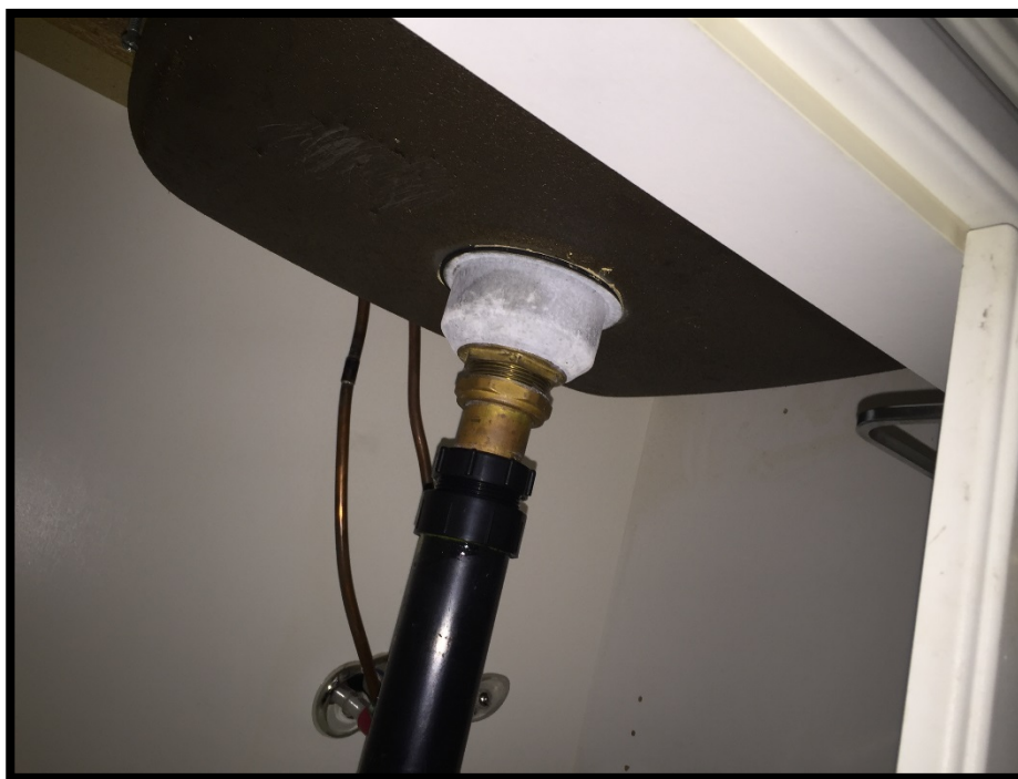
Photograph 1: Asbestos-Containing Gold Sink Undercoat.
