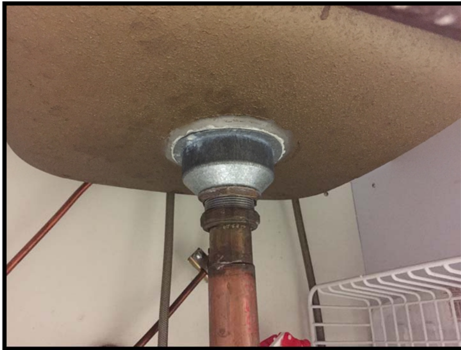
Photograph 1: Asbestos-Containing Gold/Silver Sink Undercoat.
