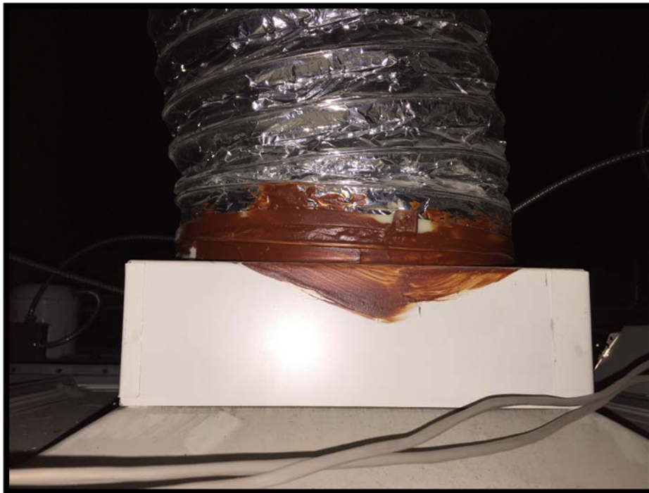
Photograph 2: Asbestos-Containing Red/Brown Duct Mastic.
