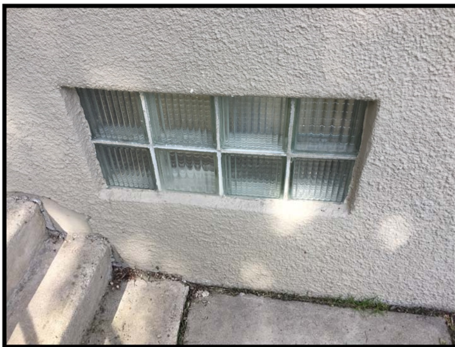
Photograph 1: Asbestos-Containing Exterior Stucco.
