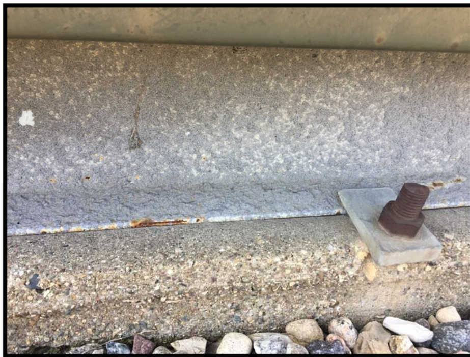
Photograph 2: Asbestos-Containing Texture Coat.
