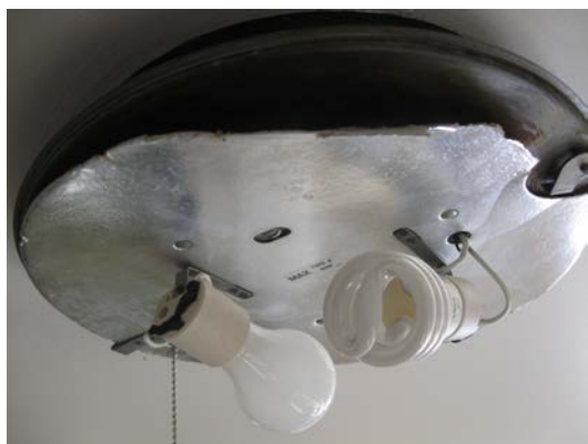
#7) Heat Shield in Light Fixture
