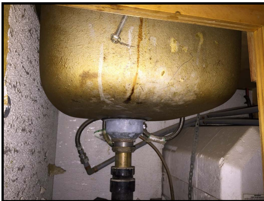
Photograph 1: Asbestos-Containing Gold Sink Undercoat.
