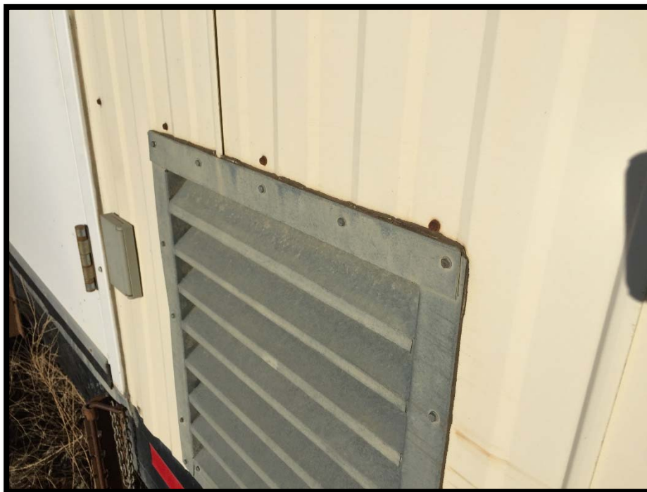
Photograph 2: Asbestos-Containing Black Building Caulking.
