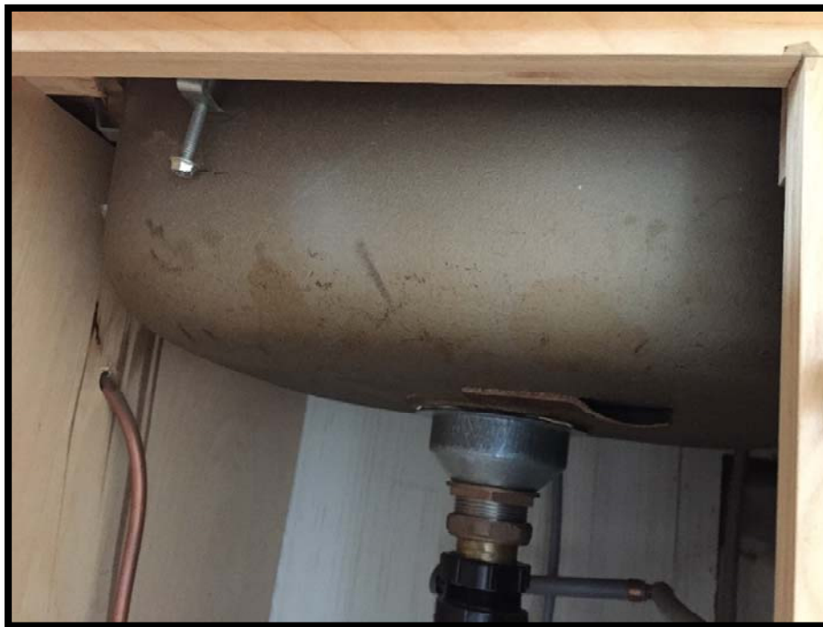
Photograph 1: Asbestos-Containing Gold Sink Undercoat.
