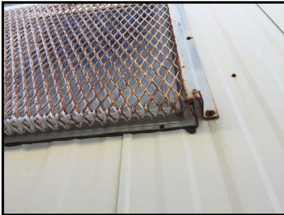
Photograph 2: Asbestos-Containing Black Building Caulking.
