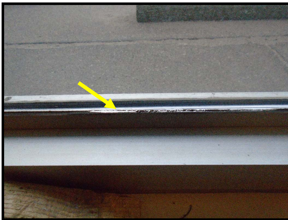
Photograph 1: Asbestos-Containing Black Window Caulking.
