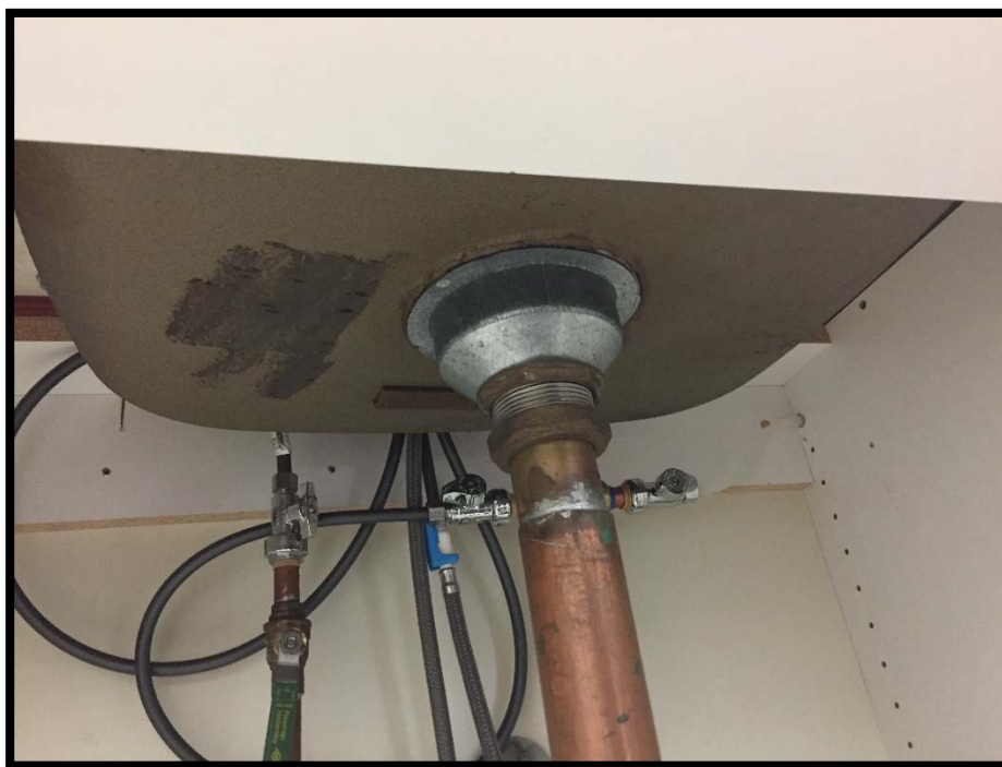
Photograph 1: Asbestos-Containing Gold Sink Undercoat.
